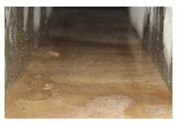
Figure 14. Plenum under bin 9 (ozone treatment) on date of shipment 2/17/2014. Note leakage on bottom and sides.
