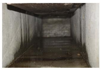
Figure 13. Plenum under bin 8 (control bin) on the date of shipment 2/17/2014. Note leakage on bottom and sides.
